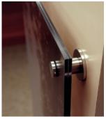
Historical images were printed onto 3Form acrylic sheets and then mounted to laminate end panels installed on the Spacesaver cantilever shelving.
